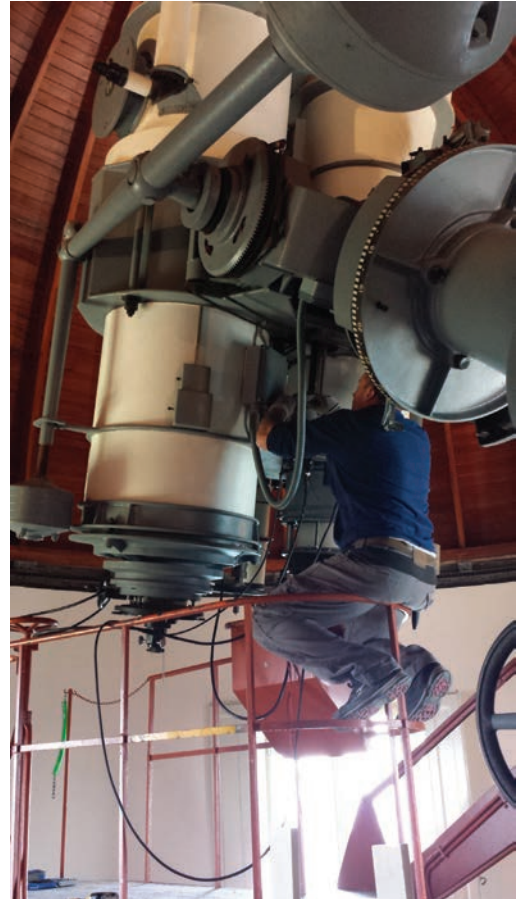
Maintenance work on the Zeiss Double Astrograph, Castel Gandolfo
