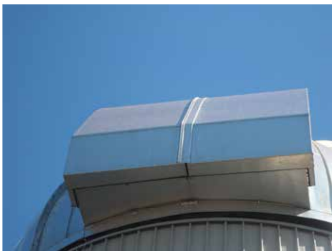
The dome slit faced south during the fire, overlooking an area of intense heat (cfr. next photograph). Note the absence of any sign of damage except for the fine layer of fire retardant (pink).
