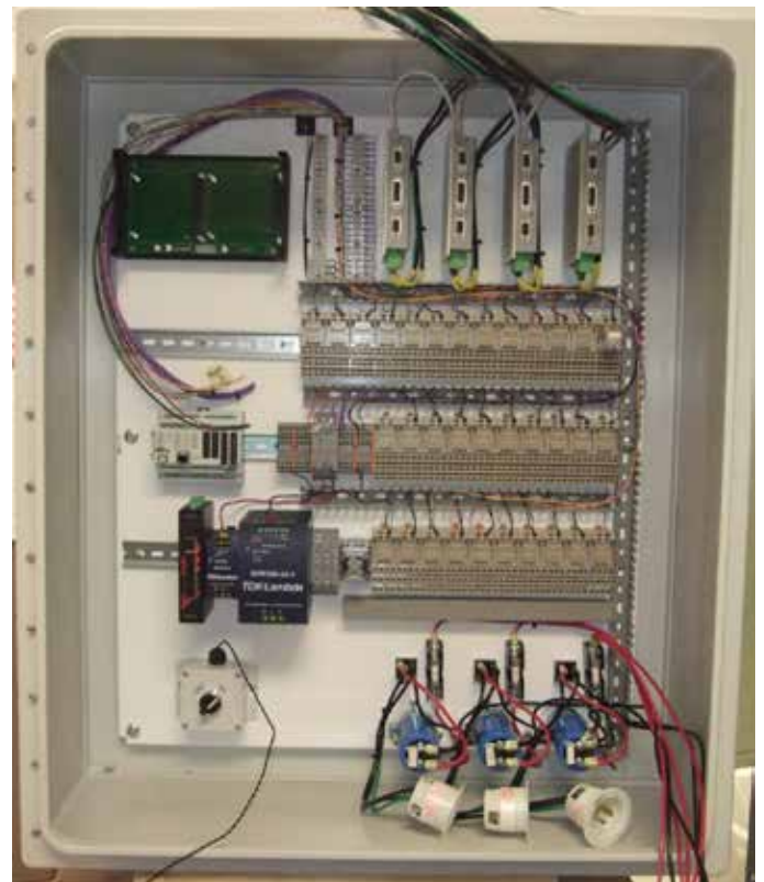
NGTCS Local Control Unit, including (clockwise from top left) the berth for the computer stack, four ELMO drive units, ladder logic relays, capacitors, fuses and power supply units, and the Arduino unit (Controllino Mega)
