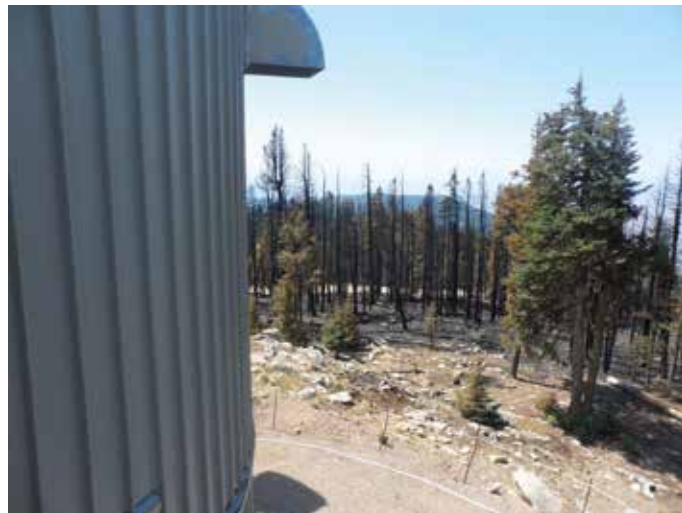
View from the SW balcony off VATT's control room towards the south-southeast. An intense blaze devastated the trees as close as 50 ft from the foot of our building
