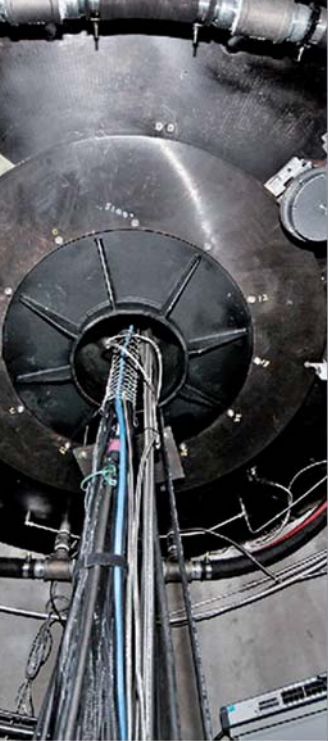
New oil return lines from the VATT azimuth bearing, from a view immediately below the telescope. David Harvey Photography
