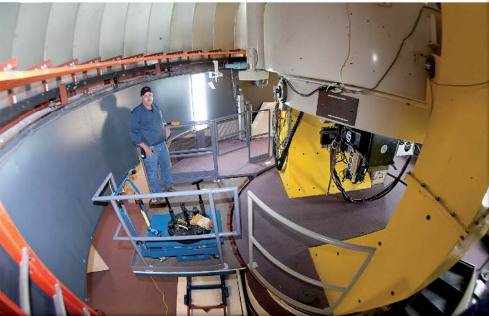
Gary Gray standing on the scissors elevator and besides the new extended decking around VATT. The Camera GUF1 hangs from the telescope. David Harvey photography
